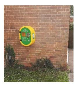
The highly visible and secure cabinet, complete with electrical connection to provide an identifying light, and heater, was funded by the Circuit and installed while our electrician was on site. With the lifesaving device inside the cabinet being provided to us as a gift from Thames Valley Heartbeat.
