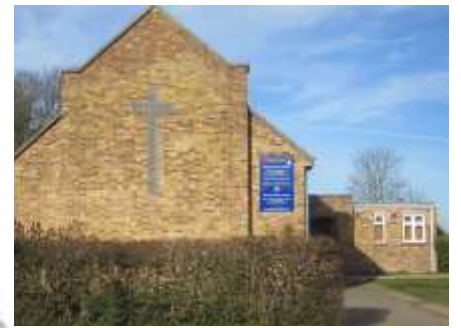
Woodthorpe Methodist Church, Edinburgh Drive
