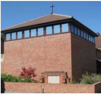
Woodthorpe Methodist Church, Clarendon Road
